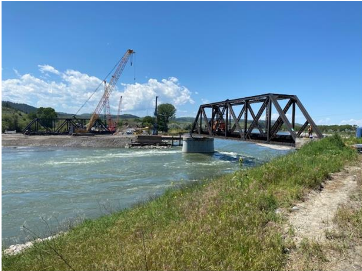
Bridge construction activity
