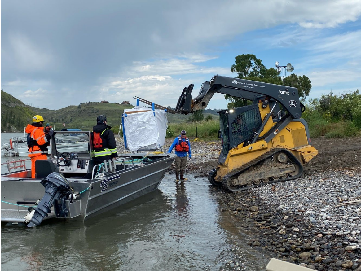
Crews unloading asphalt materials
