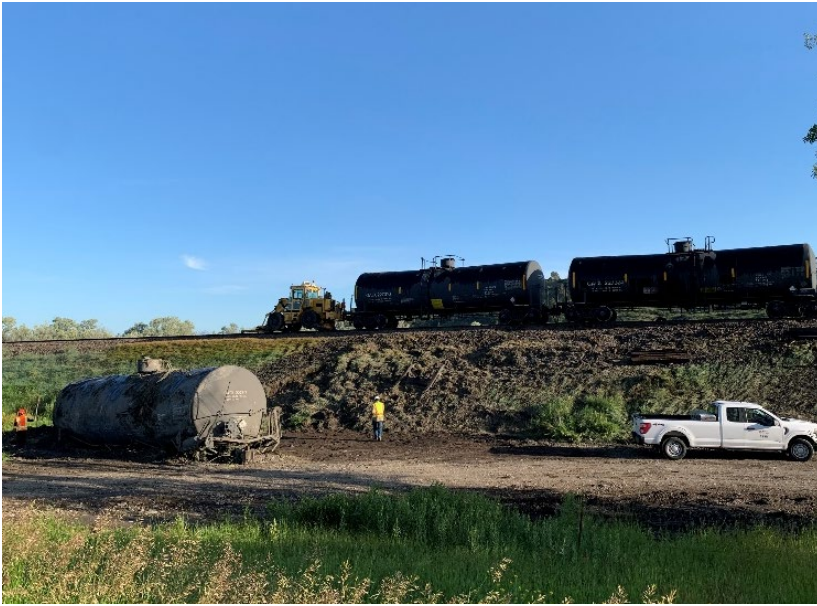
Photo of empty rail car that previously contained sodium hydrosulfide [bottom left] and the two new rail cars containing the sodium hydrosulfide.
