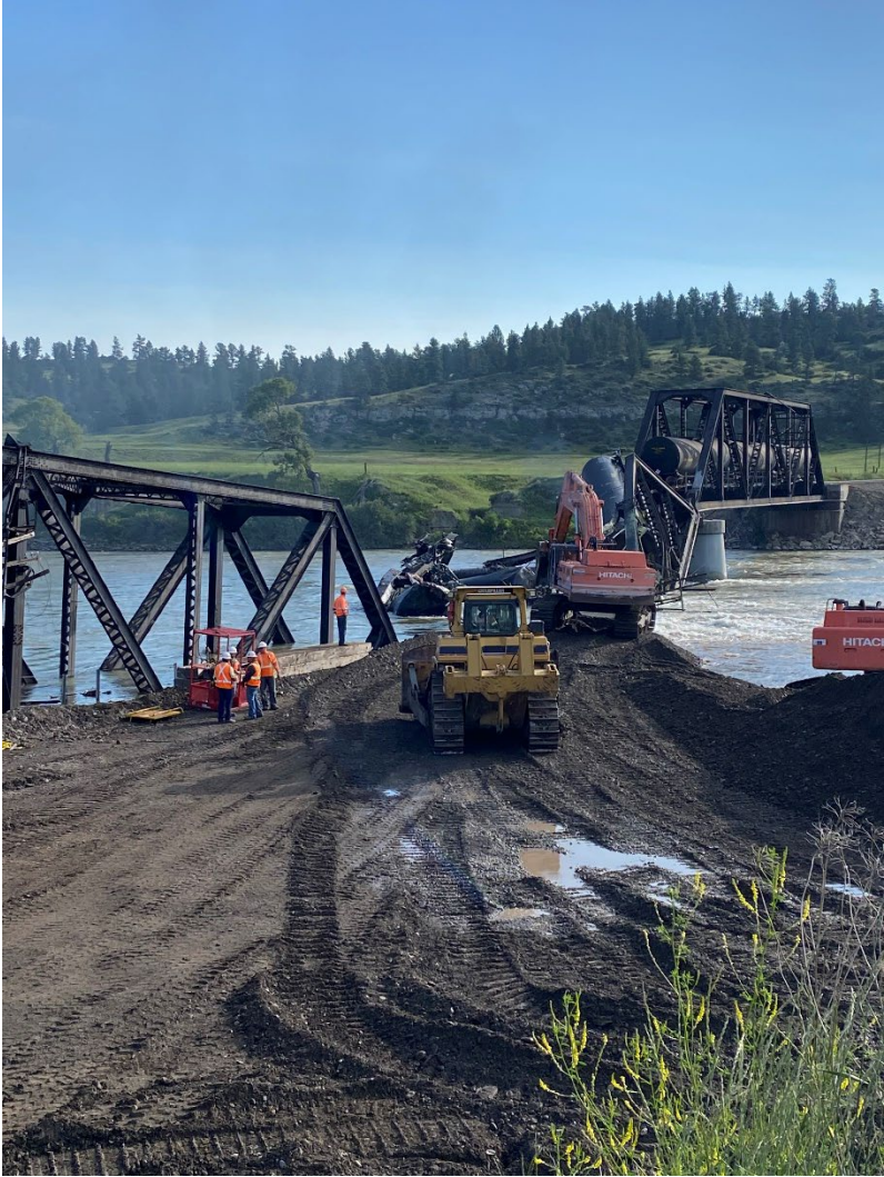
Causeway and construction equipment.
